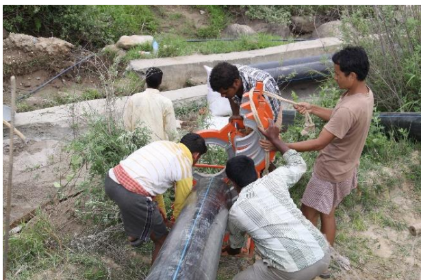
Image 4: Laying of the Pipeline
