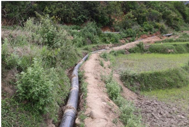
Image 2: Construction of the Siphon
