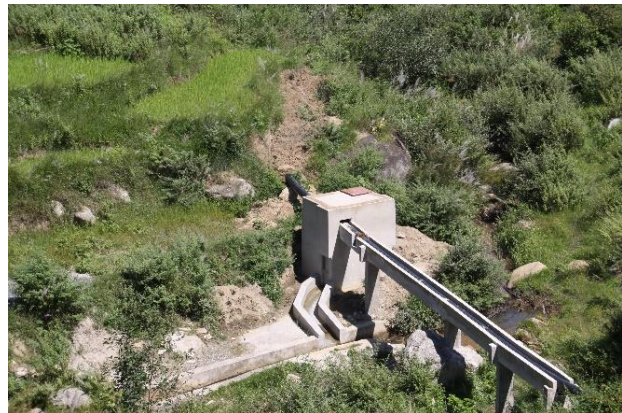
Image 3: Completed Intake Structure
