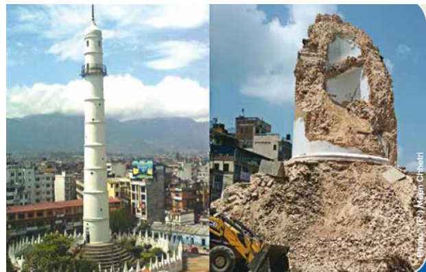
Figure 1. Dharahara (Icon of Kathmandu) – before and after the Gorkha 2015 earthquake (from GoN, 2015)
