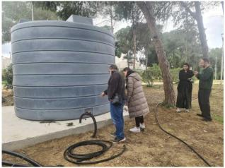
MISSION WATER CYPRUS Program, Cyprus (funded by The Coca-Cola Foundation) – in progress. Picture 4. The construction of a treated wastewater refill station for the municipal water tracks to use treated wastewater for irrigation of parks instead of groundwater.
